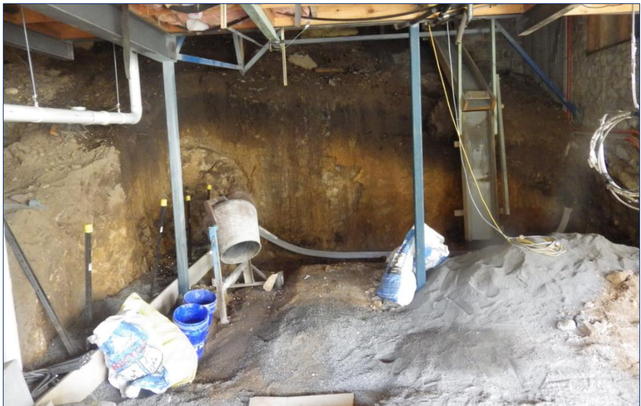
Figure 11 | Basement floor level works and excavation area (Source: Department inspection)
