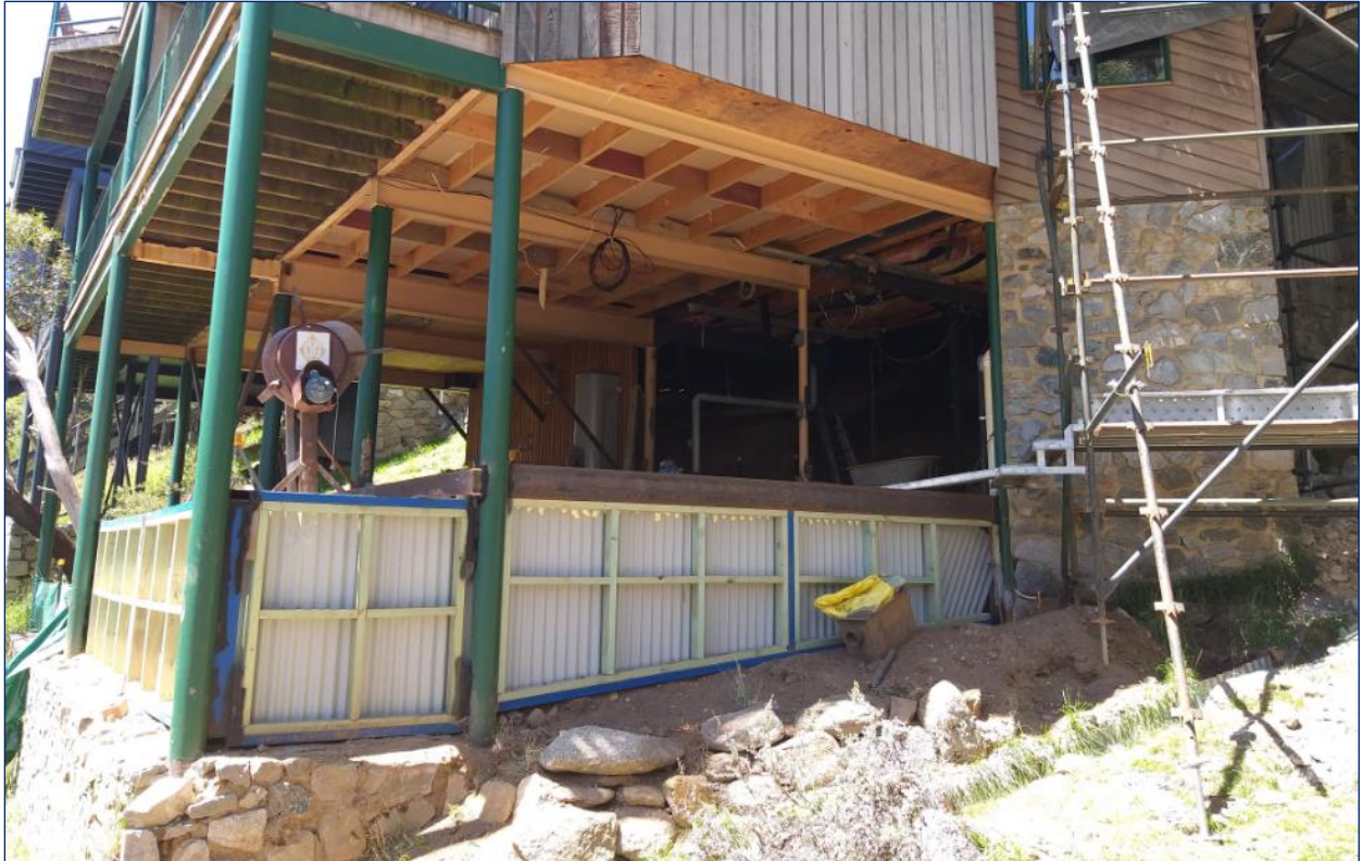
Figure 9 | Basement floor level works (Source: Department inspection)
