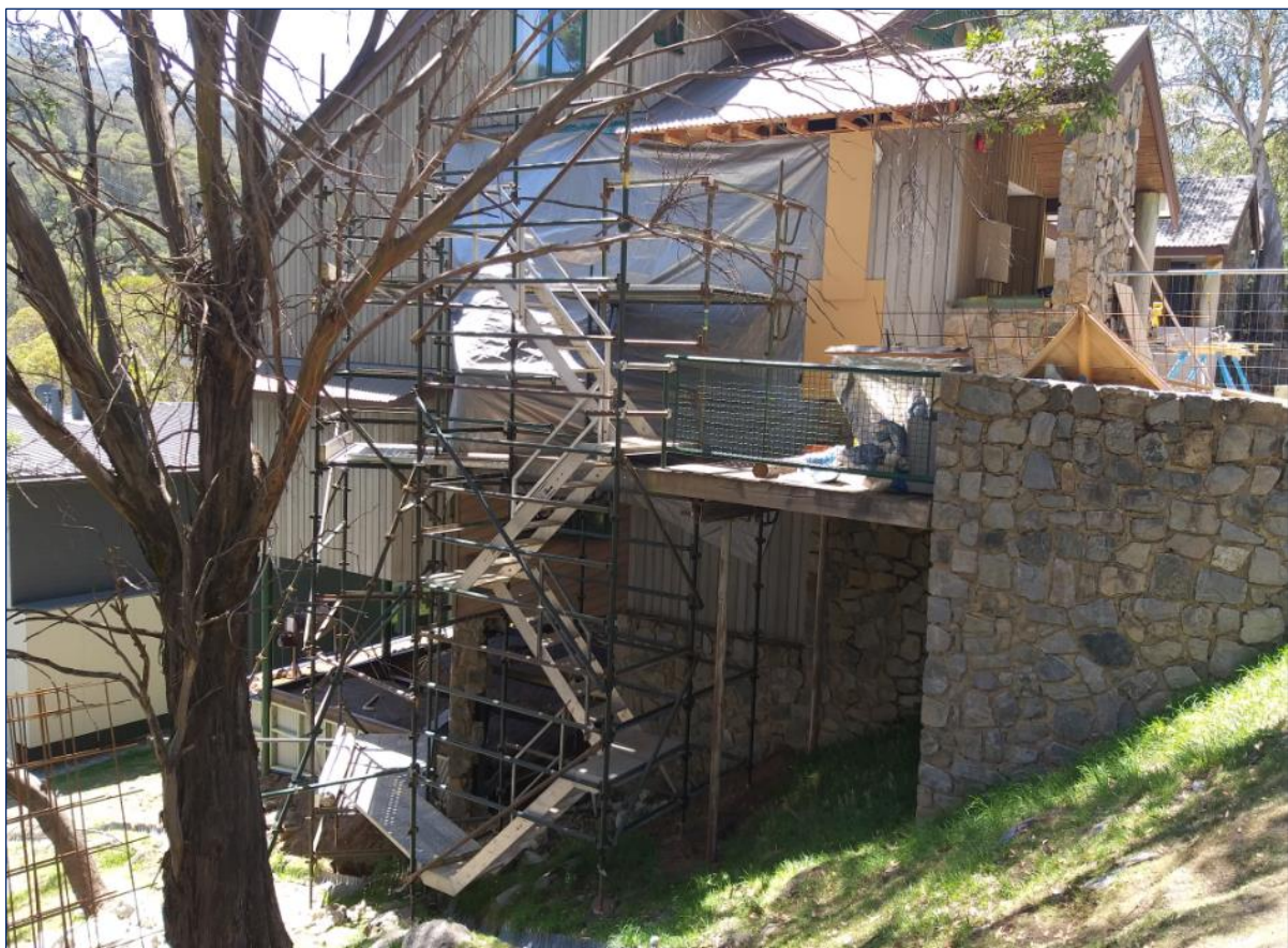
Figure 3 | Construction works during February 2020 (Source: Department inspection)
